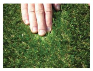
When all jointing and positioning has been completed fit the ground pins to secure the grass from lifting due to wind or trafficking. Simply hammer the pins in around the outer edges of the layout at 800 mm centres. Ground pins must always be used to secure the grass. When installing the pins remember to widen the grass so the pin traps as little of the grass as possible underneath.
