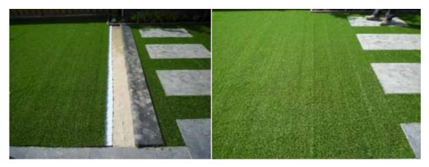
Carefully open up the artificial turf little by little and then press firmly. Make sure there are no blades of grass trapped in the joint. Press again by walking across the artificial turf.
