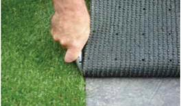
If you have to make a joint across the stitching, make sure you use a straight edge and cut the artificial turf along this edge. You need to do this on both sides. After cutting two pieces of artificial turf, lay these beside each other for joining as explained later.
