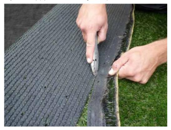
When joining several pieces/rolls of artificial turf next to each other, make sure both sides are cut close to the fibre stitching. Lay the pieces alongside each other to have an opening of about 3 - 4 mm. Never put the pieces next to each other too tight.
