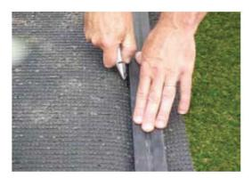
Make sure you always have the stitching and direction of the fibre (nap) in the same direction. Never join across the stitching and along the stitching together.
